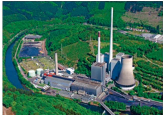
The power generation plant in Werdohl-Elverlingsen
