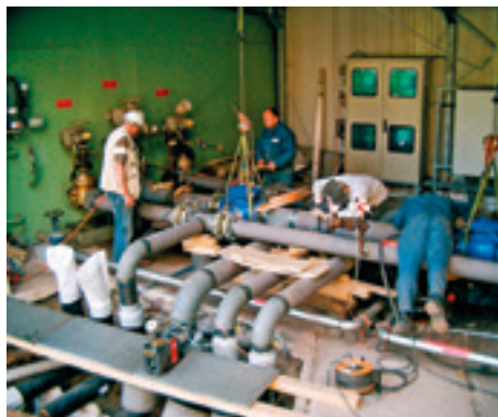
Embedding work between Tank 1 and Tank 2
