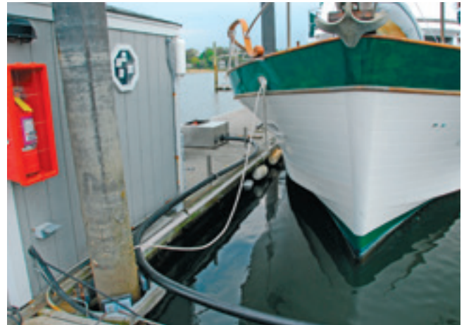
Connecting it to the fuel dispensers
