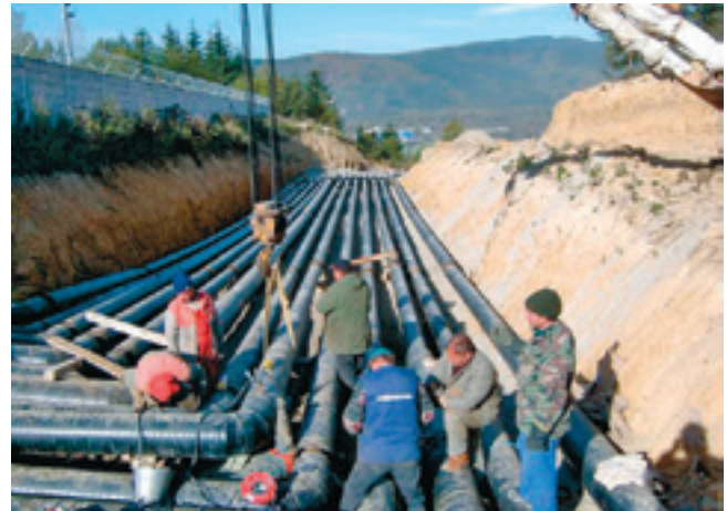
Fitting the external protective sheathing to the BRUGG-STAMANT® safety piping
