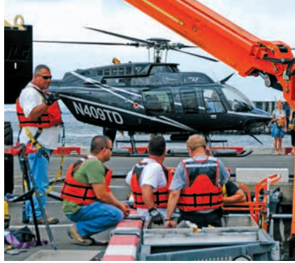
Installation work with no interruption in flight services
