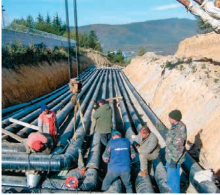
Installing the outer pipe casing BRUGG-STAMANT® Safety Pipe
