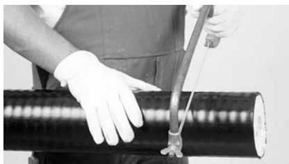
2 Cut the casing pipe with saw.
