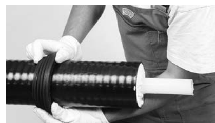
6 Install the wall sealing ring.
