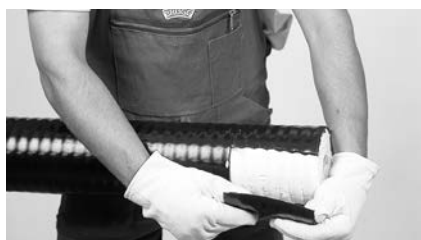
4 Peel off the casing.
