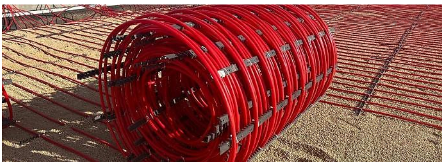
RAUMAT automated prefabricated mats install up to 85% faster while reducing labor by up to 75%. © REHAU
