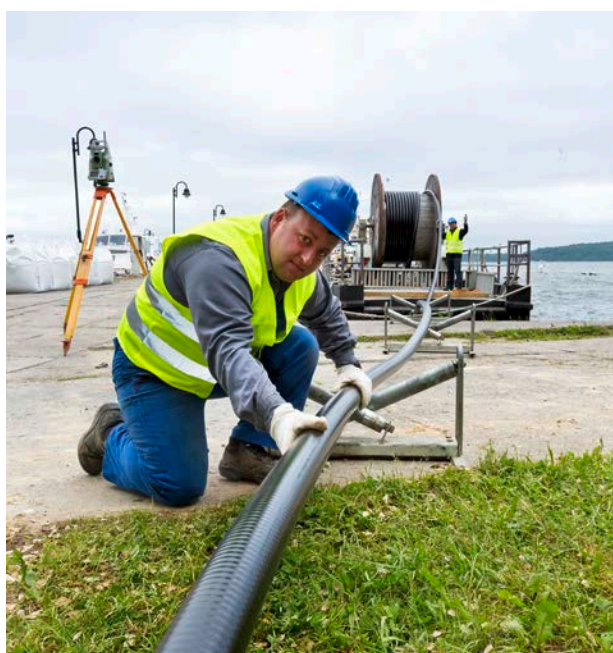
Figure 2. Laying of flexible-stainless steel pipe.
