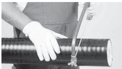
2 Cut the casing pipe with saw.
