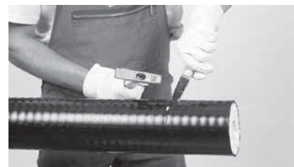
3 Split the casing pipe with knife. Note: Don't damage the carrier pipe!
