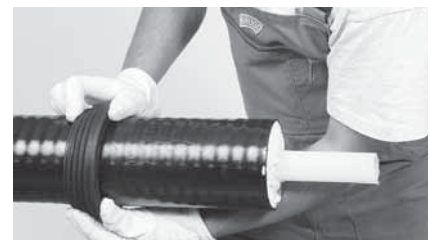
6 Install the wall sealing ring.
