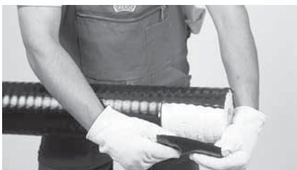
4 Peel off the casing.
