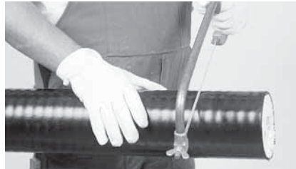
2 Cut the casing pipe with saw.
