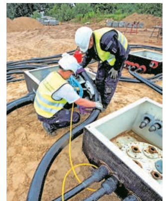
Bending the piping
