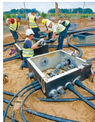
Laying the filling line
