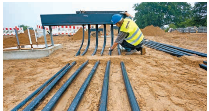
Laying the piping to the future petrol pumps
