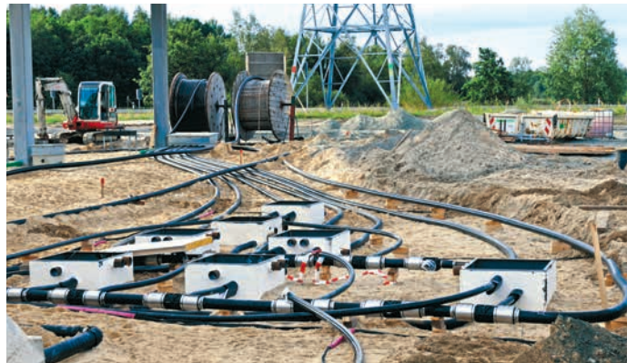
Laying the filling pipes directly off the drum
