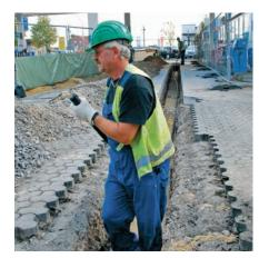
FLEXWELL®-LPG - flexible pipe system for automotive LPG in service station constructions: DN 25-DN 50, PN 25
