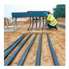
SECON®-X - double walled flexible fill pipe for automotive fuels in petrol station constructions: DN 25-DN 100, PN 10
