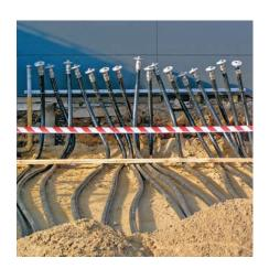
PETREX®-CNT - Flexible, singlewalled pipe system with stainless steel inner pipe as delivery pipe for fuels in petrol station constructions: DN 25-DN 80, PN 10
