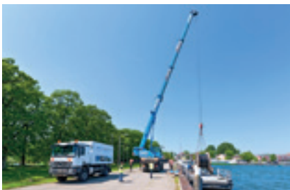
Transferring the pipe drum to the barge
