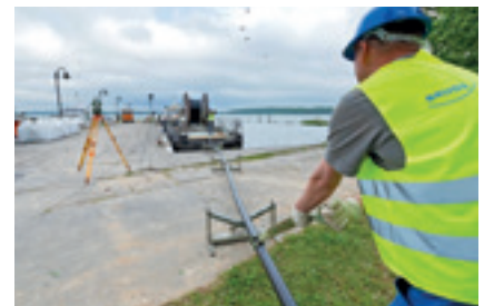
Unrolling the pipe
