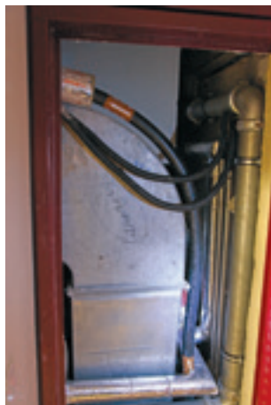
Despite tight conditions in the building: pipe laid without molded parts
