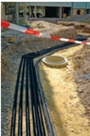
Laying the pipe in the trench
