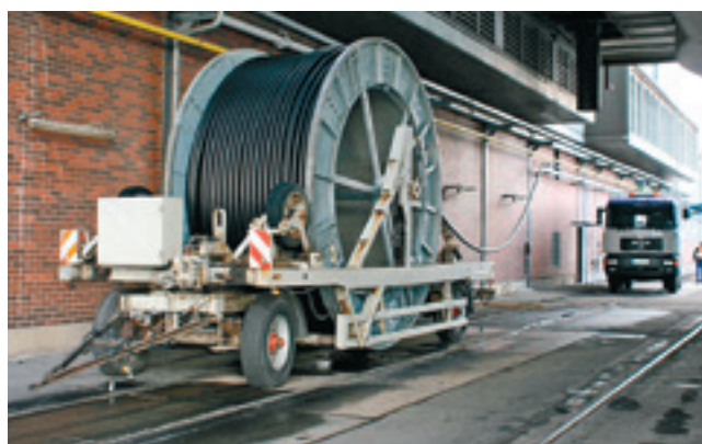
Laying the piping directly off the reel onto the cable racks
