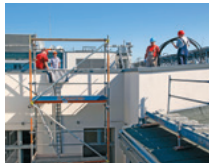
Thanks to its excellent flexibility the FLEXWELL® Safety Pipe can be laid with ease across the roof, changing direction several times.
