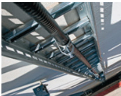
Simple fixing of the FLEXWELL® Safety Pipe with system technology (anchor and cable saddle brackets).
