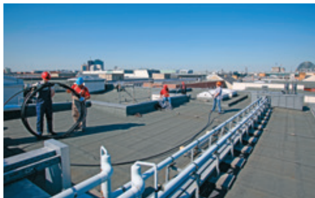
Laying the FLEXWELL® Safety Pipe on the roof.
