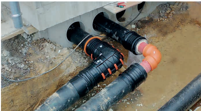
Figure 3. Clip-Flex L-shrouds with deviation during pipe installation 160/250 mm pipe joint
