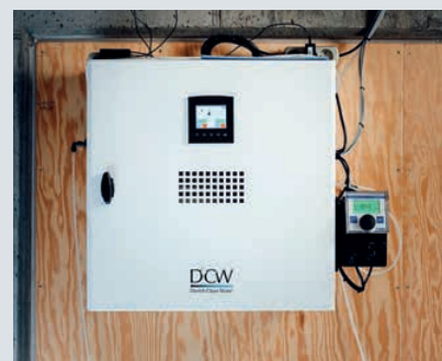
The generator from Danish Clean Water disinfects drinking water efficiently, killing dangerous bacteria such as Legionella
